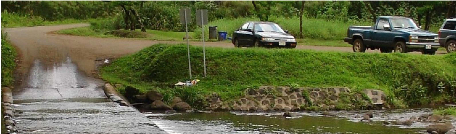
Figure 6: Photograph of the Keāhua Stream Ford pre-flood, view to East (adapted from Powell et al. 2014) The ford is lightly eroded but intact, and the Post-Contact wall is visible to the right, with the parking lot behind it on the rise.
