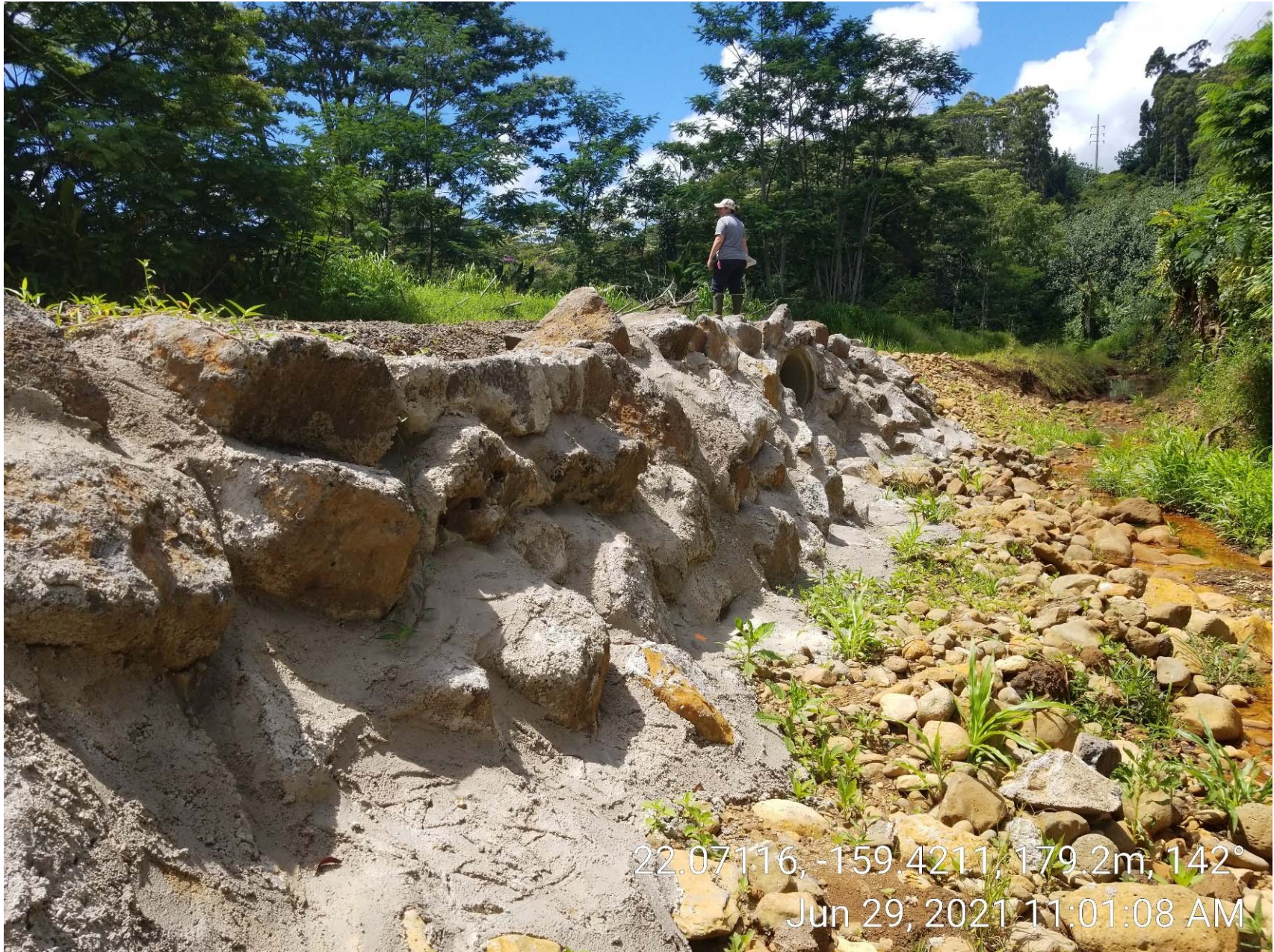
Figure 11: Photograph of the concrete and basalt boulder road crossing erected (as repairs) at the New Crossing
